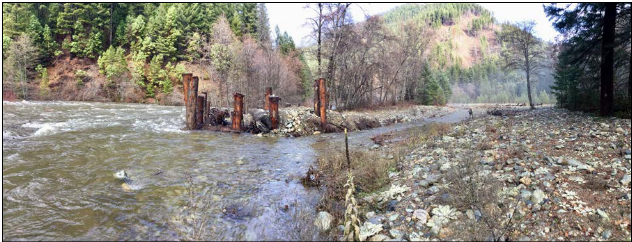
Image 19: Kelly Bar Engineered Log Jam post-implementation. January 2021.
