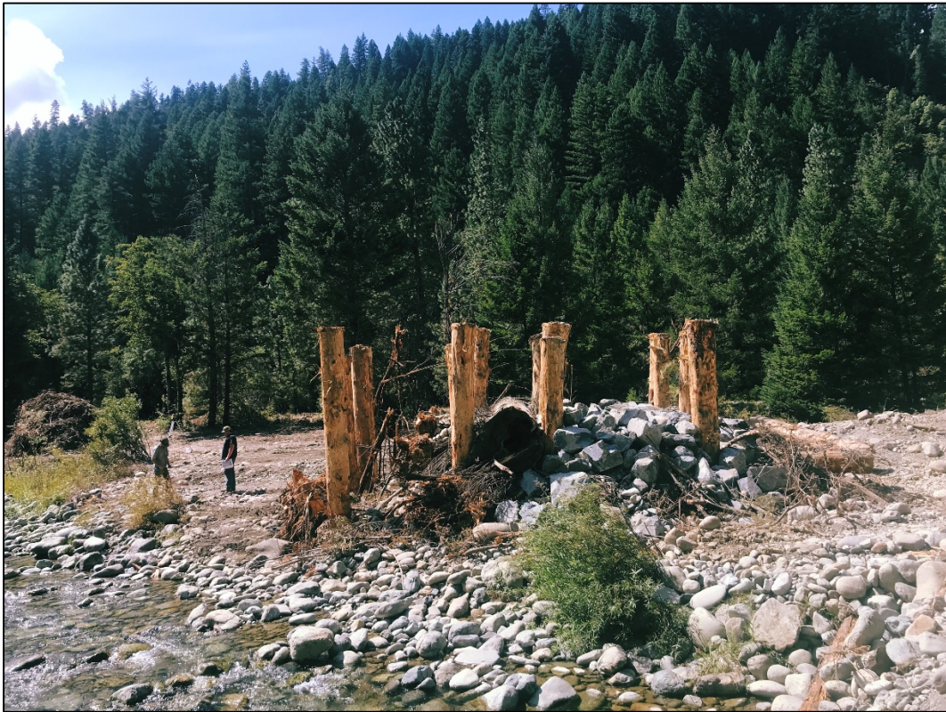
Image 6: Mid-Bar engineered log jam completed. Summer 2019.
