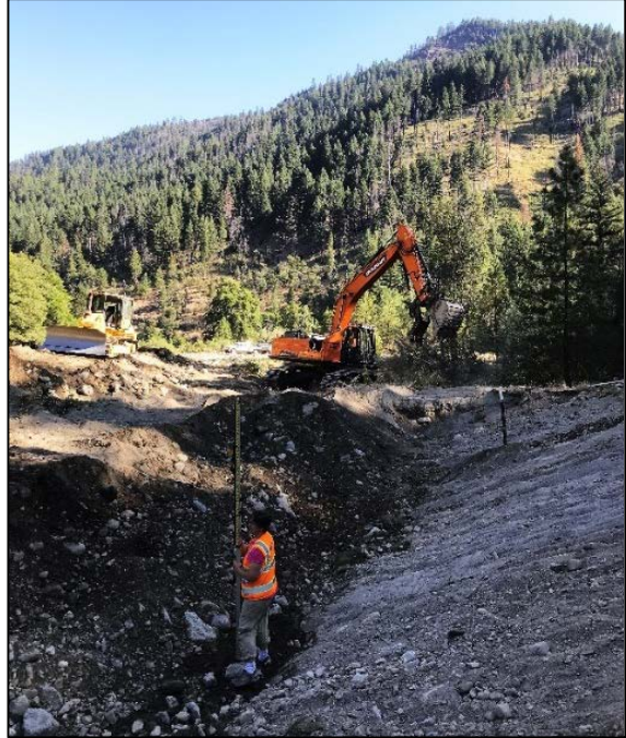
Image 5: Seasonal Channel construction. Summer 2019.
