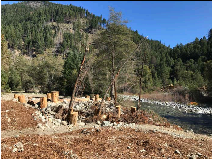
Image 27: Recently completed Back-Bar Channel. October 2019.
