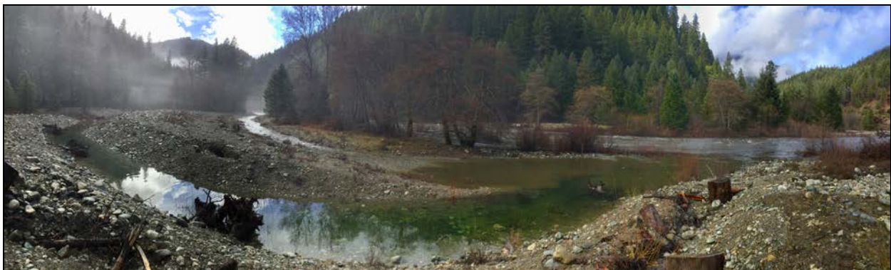
Image 11: Kelly Bar post-implementation showing Seasonal Channel on left, Overflow Channel at center, and Kelly Bar Alcove on right. January 2021.
