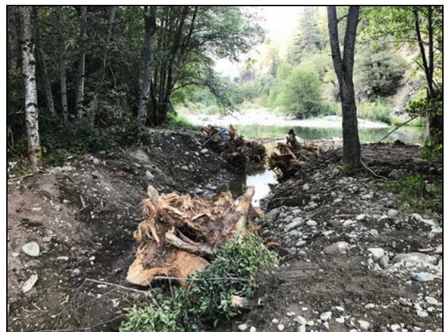
Figure 26: Just completed West Bar Alcove. September 2019.
